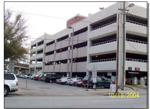
Evaluated appearance and condition of parking facilities.
