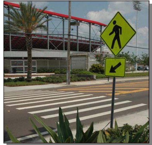
Roadway changed from a four-lane undivided cross section to a two lane divided cross section that improves pedestrian safety and traffic operations.
